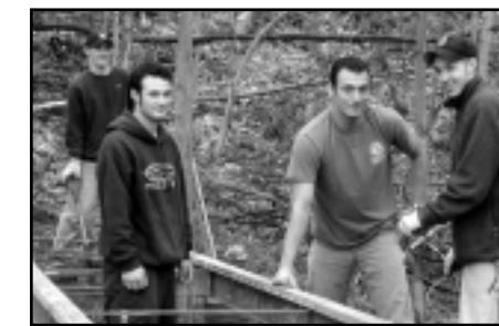
Planning the bridge.
